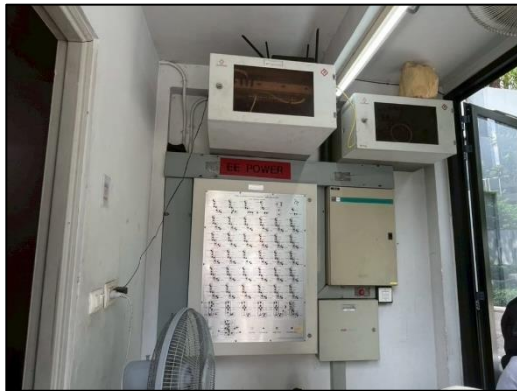
Fire Alarm System Graphic Annunciator
