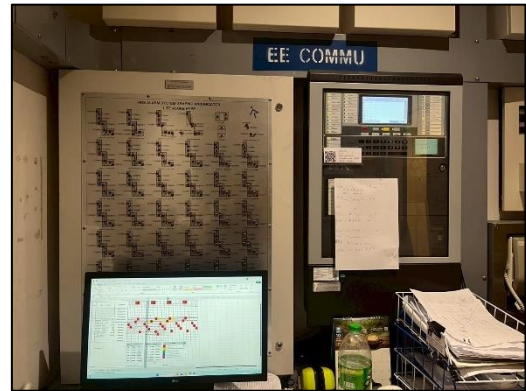
Fire Alarm Control Panel
